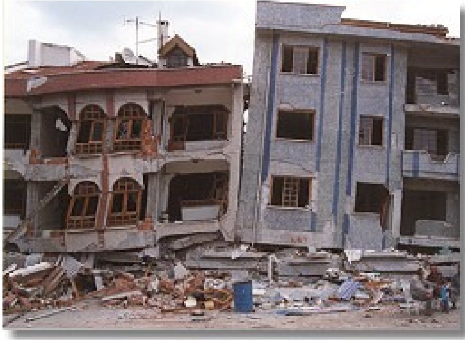
Figure 1. Building pounding (New Zealand, 2009).
